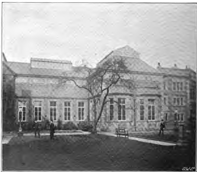
4. OUTSIDE VIEW OF READING ROOM AND REFERENCE LIBRARY, CARLISLE.
